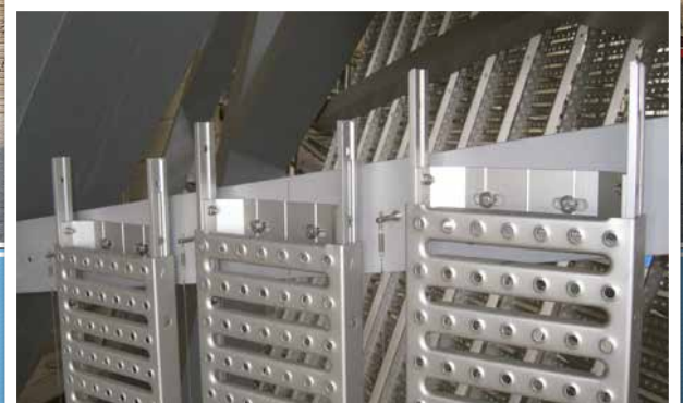
Hollo-Bolts connect the cladding panel brackets
